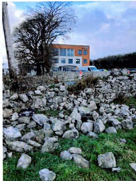
Photos 4 & 5: Damage caused to road wall after recent accident, November 2024
